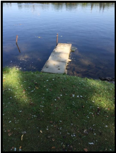
Figure 13. Degraded/absent vegetated buffer zones at site BPC.
