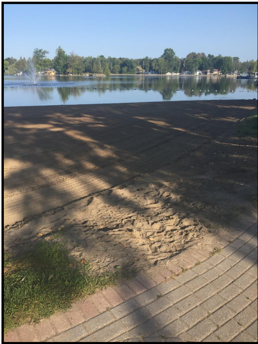
Figure 15. Evidence of stormwater pooling in the upshore area.
