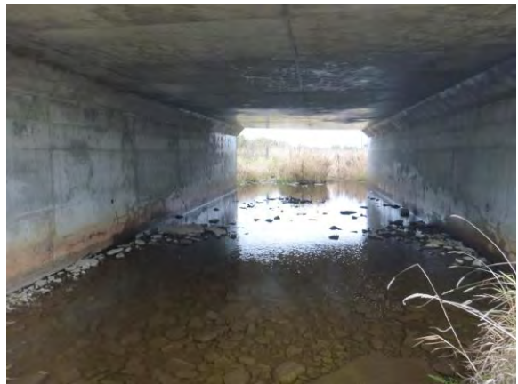
Upstream end of Culvert
