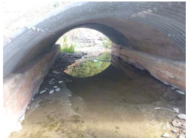
Upstream end of Culvert
