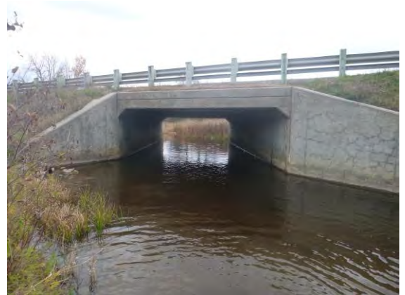
Upstream end of Culvert
