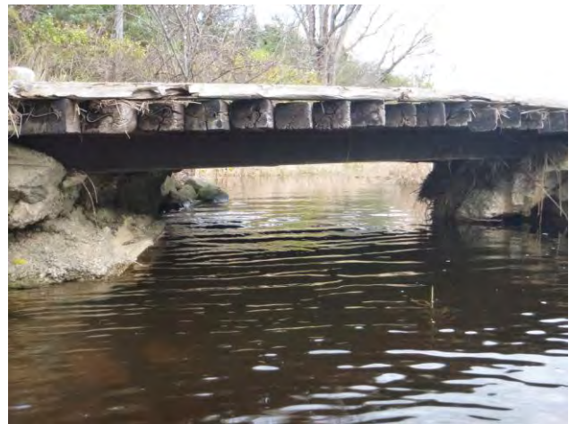
Upstream end of Culvert
