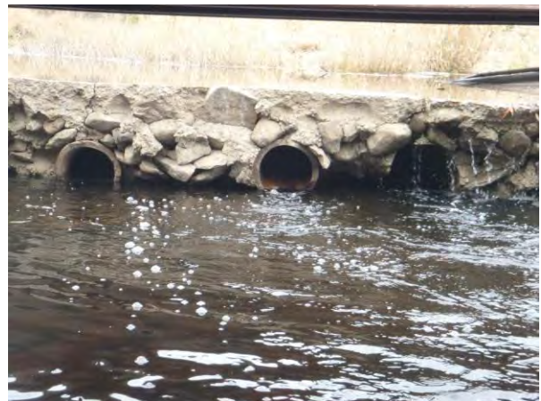
Looking Upstream under Bridge
