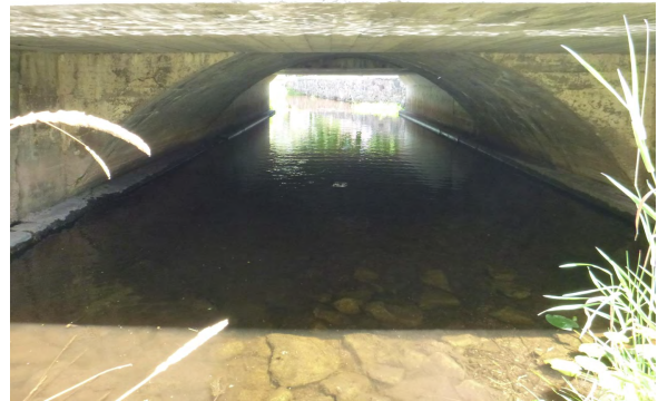
Upstream end of Culvert
