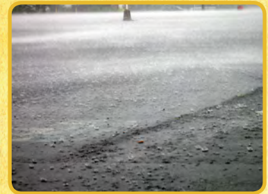
Hard, impervious surfaces channel rain and snow into water bodies. This runoff can carry high amounts of nutrients and other pollutants.
