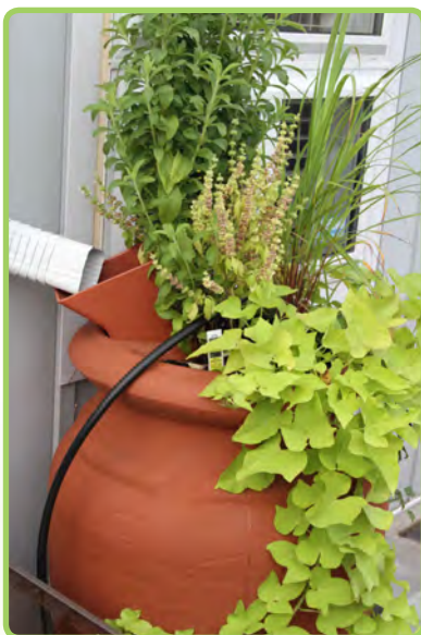
The downspout empties into the top of the barrel, which features a small garden.
