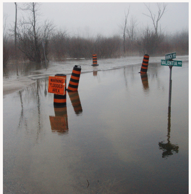
Road closure due to extreme flooding.
