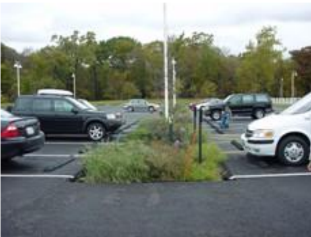
Bioswales can be used to manage and treat stormwater runoff from larger developments and parking lots. These bioswales are designed to filter pollutants, regulate flows and increase infiltration.
