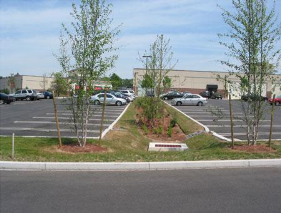
Bioretention at Evergreen Walk mall in South Windsor. For details about this project from the CT LID database, visit http://clear.uconn.edu/tools/lid/pdf/CT0012.pdf
