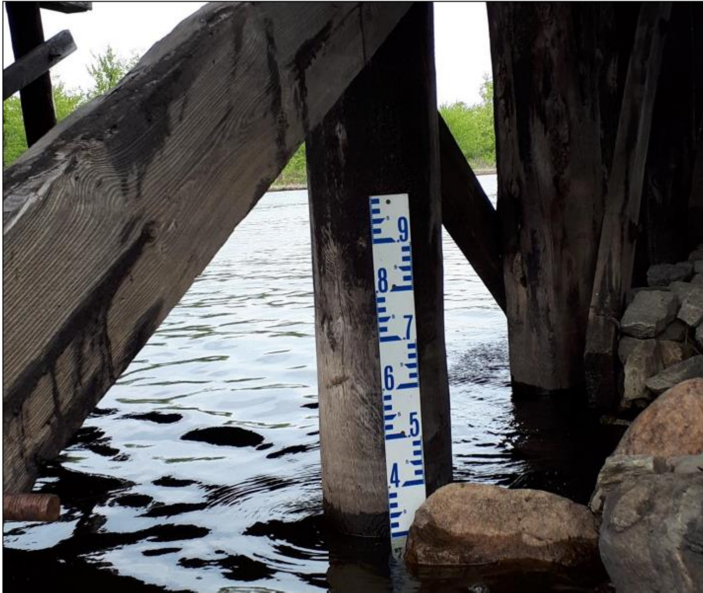
[Lake level monitoring gauge at the 'narrows', Kirkfield Road bridge, May 25, 2021]
