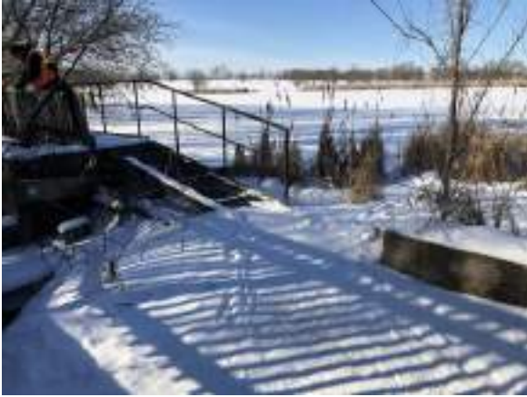
Top of Dam
