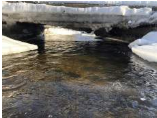
Upstream Looking in Culvert
