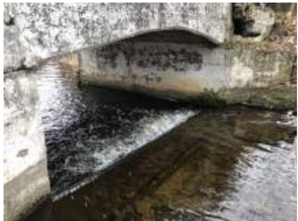
Upstream looking in culvert
