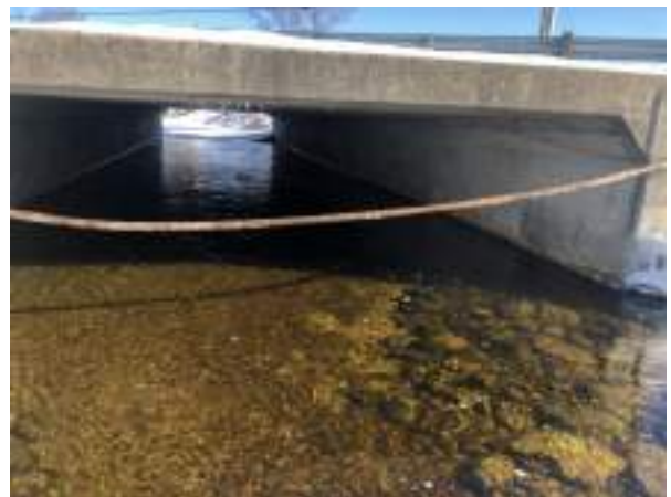
Looking in culvert from Downstream Side
