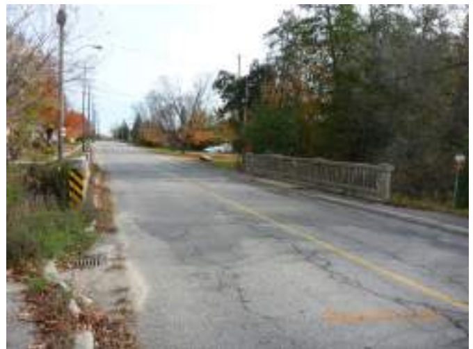
Upstream End of Culvert
