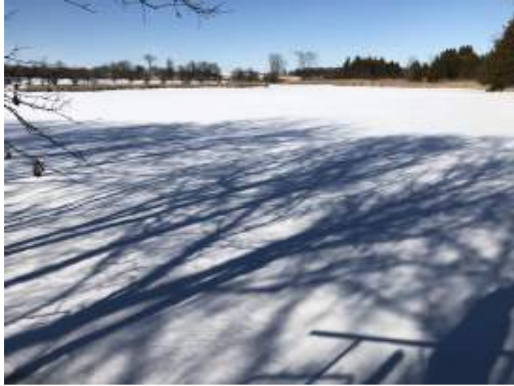
Top of Dam looking upstream
