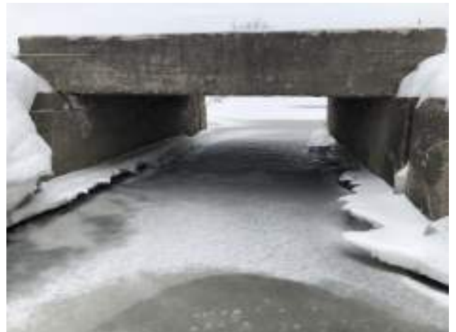
Upstream Looking into Culvert
