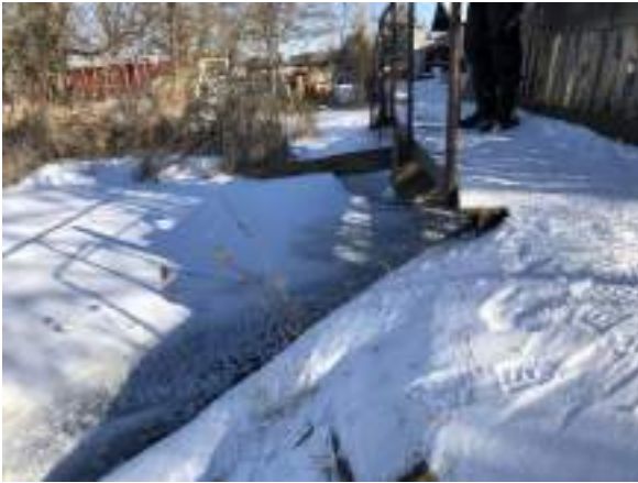
Top of dam
