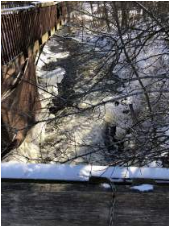
Top of Dam looking Downstream
