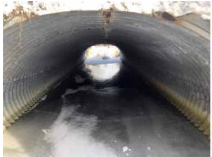
Upstream End of Culvert
