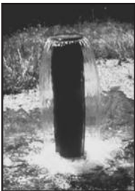
Flowing well that is not controlled.
