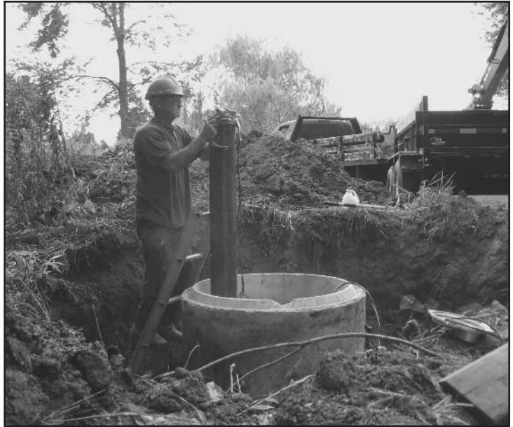
Well upgrade in progress.
